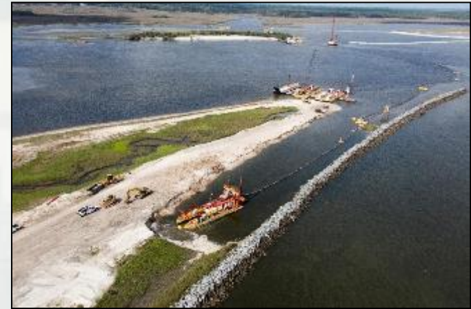
Relocation/Reconfiguration of the Mile Point Training Wall
